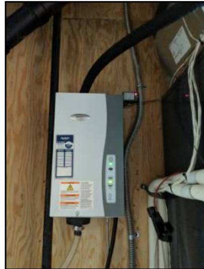
humidifier installed on the main level unit.
